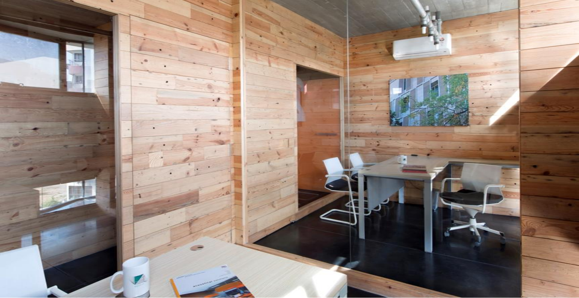
01. ZERO WASTE- 'SHUTTERING WOOD PARTITIONS'
