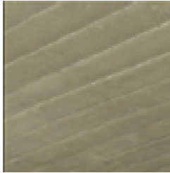
FORM FINISHED CONCRETE
