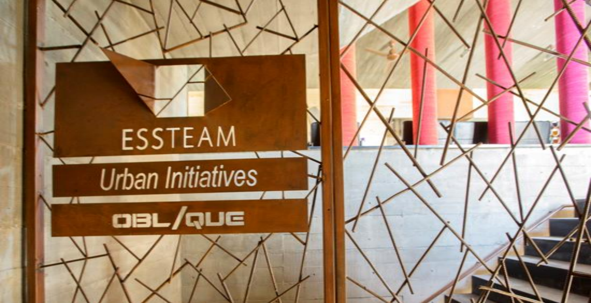
01. ZERO WASTE- 'WASTE REINFORCEMENT BARS RAILING'
